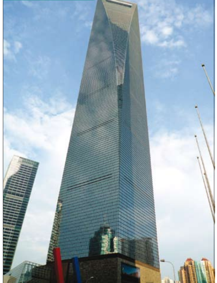
Shanghai World Finance Center: New glass, factory application
