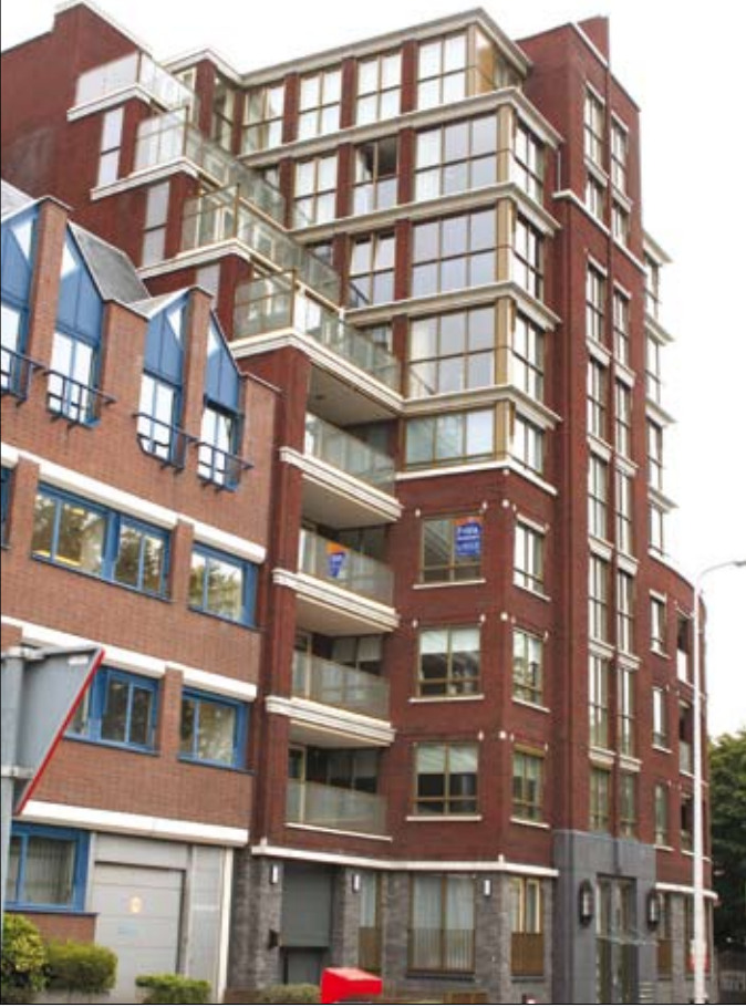
Metropole Building, The Hague: Existing glass, on-site renovation & protection
